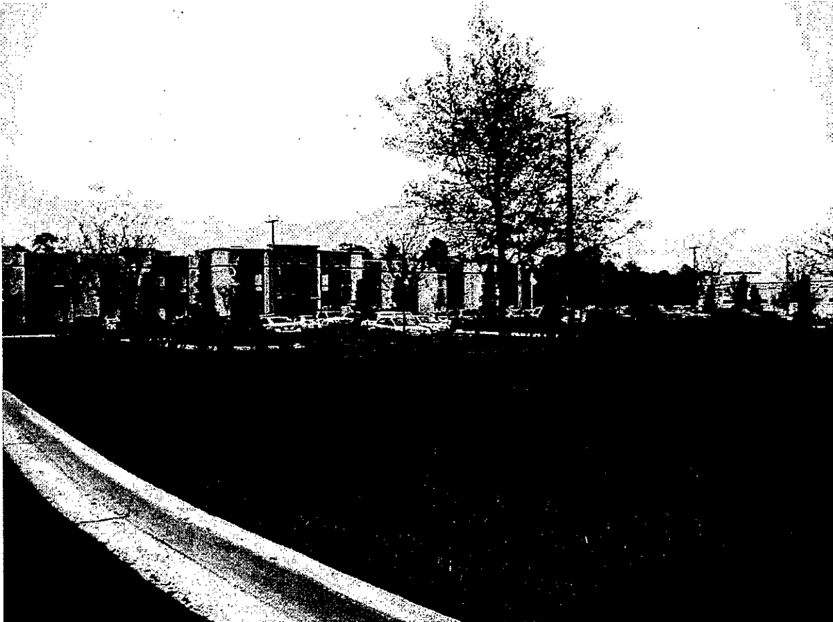
View of newly constructed building.
